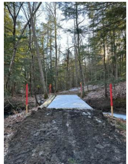
With the base pallet in place, it now needed the deck removed. Then pressure treated lumber will be installed as the bridge decking.
