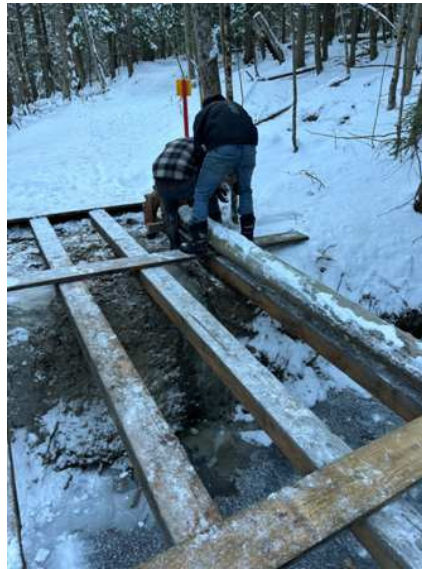
First the removal of the old decking, then the pressure treated deck is put down. Side bumpers are added for safety.
