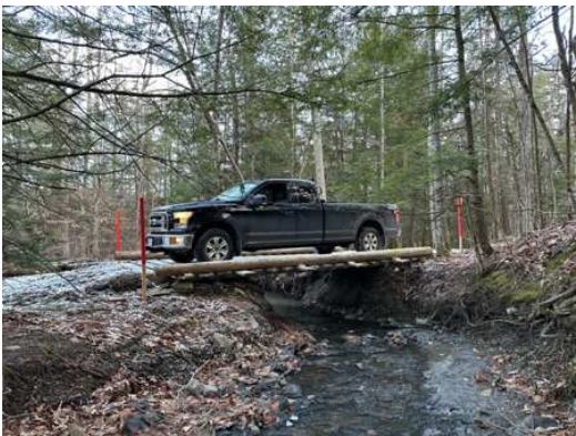
The new bridge passes truck inspection.
