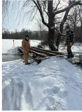
Matt Lord, Gerry Lenseith, and Brian Buchardt strip off old decking of the Long Road bridge on trail S72.
