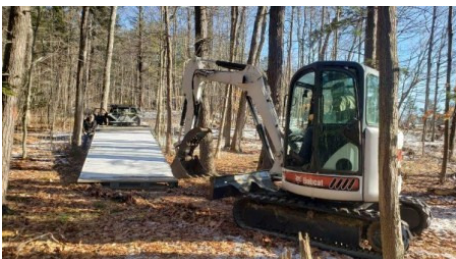
S73 - Maple Inn Trail Culvert tubes used to be here. Washed out over the summer, it was decided to replace the culverts with a bridge.
