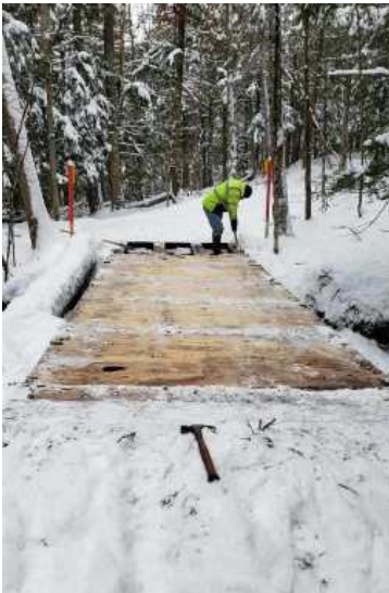
First the removal of the old decking, then the pressure treated deck is put down. Side bumpers are added for safety.
