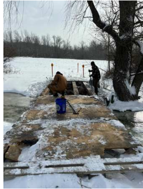
Matt Lord, Gerry Lenseith, and Brian Buchardt strip off old decking of the Long Road bridge on trail S72.
