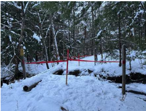
S73 - Maple Inn Trail Culvert tubes used to be here. Washed out over the summer, it was decided to replace the culverts with a bridge.
