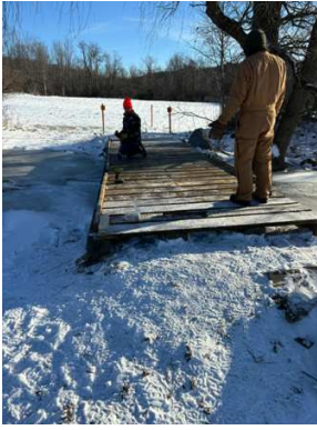
Matt Lord, Gerry Lenseith, and Brian Buchardt strip off old decking of the Long Road bridge on trail S72.
