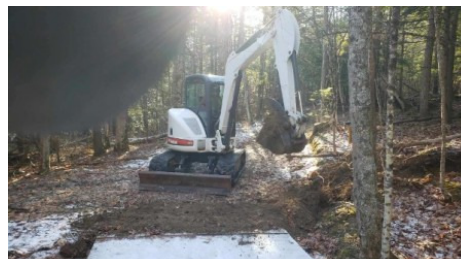
With the base pallet in place, it now needed the deck removed. Then pressure treated lumber will be installed as the bridge decking.
