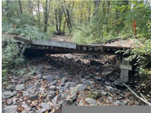
Collapsed bridge on Montgomery club trail #456 on Calovic property requires replacement frame. Photos by Gerry Lenseth.
