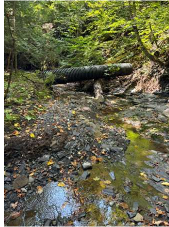
Numerous culverts were washed out during the summer and need replacement. Photos by Matt Lord.
