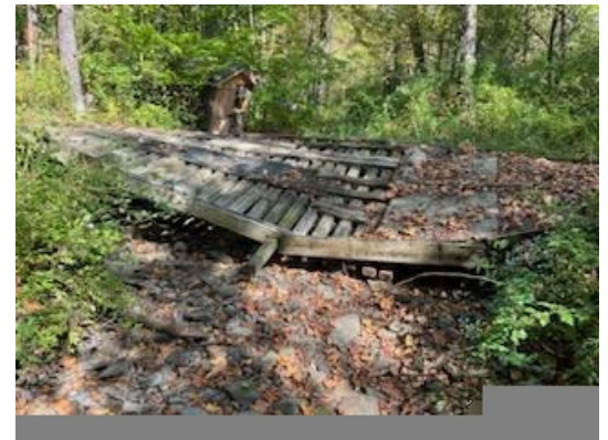
Collapsed bridge on Montgomery club trail #456 on Calovic property requires replacement frame. Photos by Gerry Lenseth.
