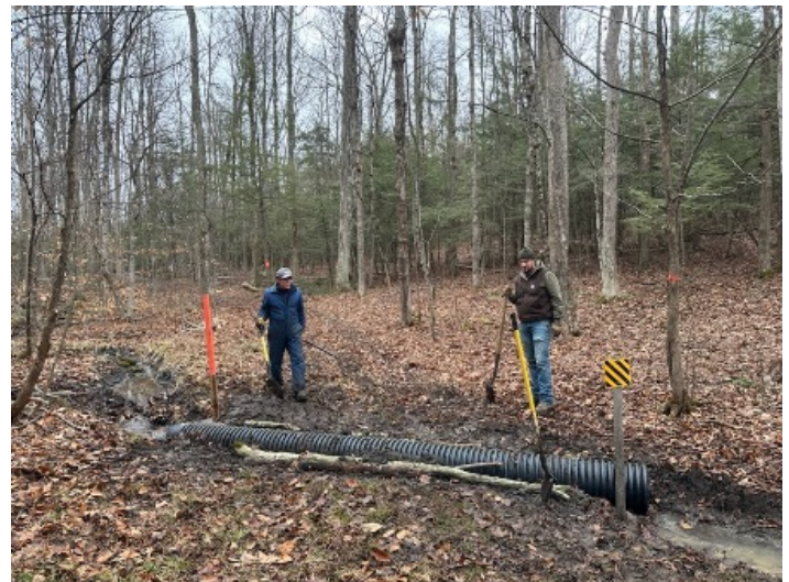
Culvert installation.
