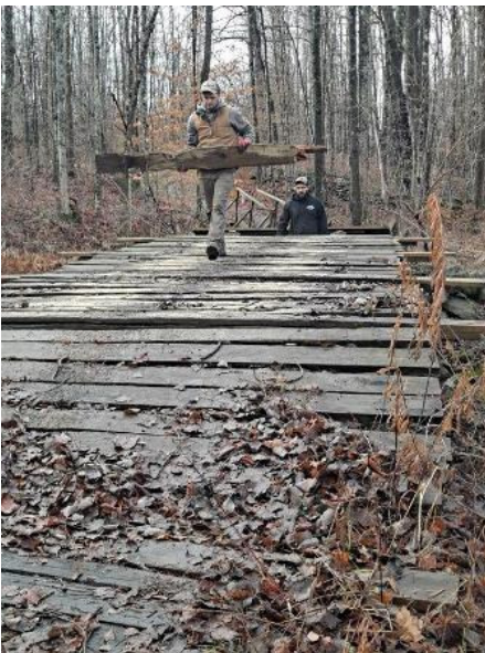
Trail Boss Tyler Walters and crew procured materials, re-decked, and also repaired the railings of the Romer bridge on C7E near Esperance. Photo by Tyler Walters.
