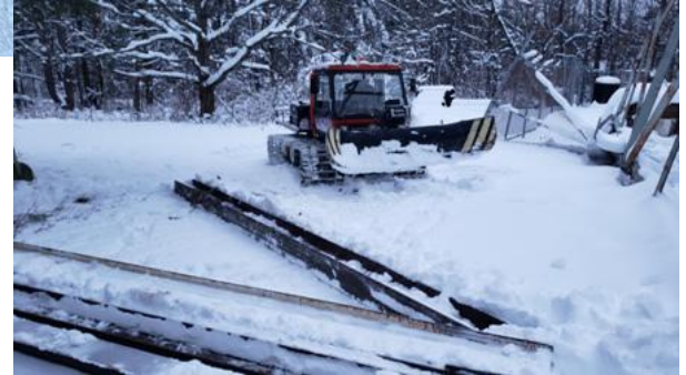
Matt Lord uses PB070 to haul out the I-beams.
