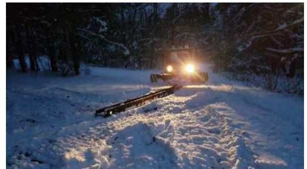
Extracting bridge I-beams for Mariaville C7B bridge.
