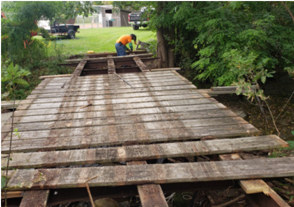
Deck partially removed-Justin Bates welding stiffeners for the excavator to grab.
