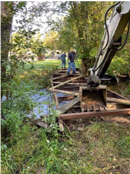
Deck partially removed-Justin Bates welding stiffeners for the excavator to grab.
