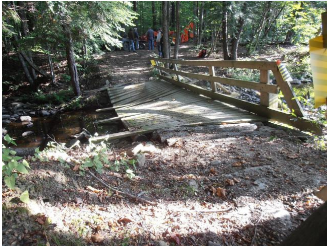
With the downstream railing removed, the damage to the bridge on C7B can be seen.
