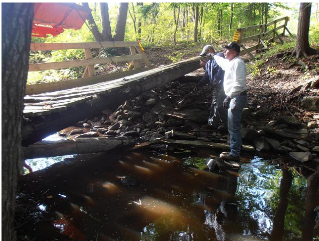
Tom Rulison helps guide the new beam under the bridge.
