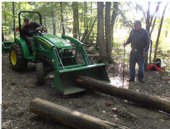
Landowner Mark pushes one of the new main beams into position with his tractor as trail boss Jerry Schoening looks on.
