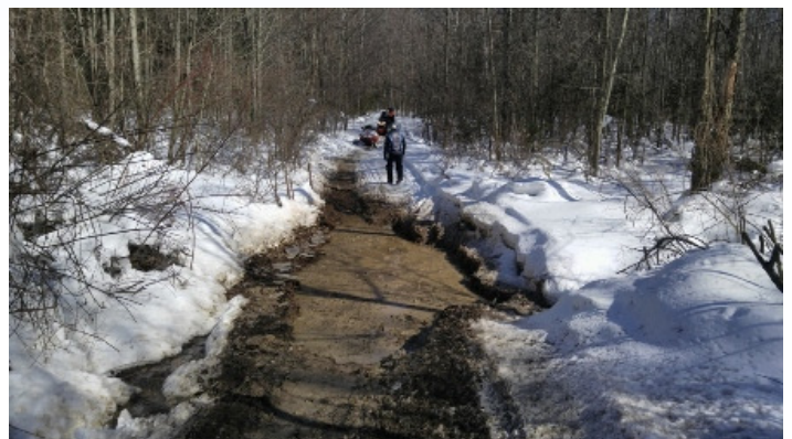
Future location for a badly needed culvert tube.
