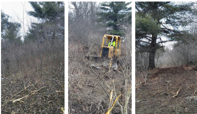
Before, during, and after, Brian Buchardt uses a dozer to open up an overgrown area for the rerouted C7B.
