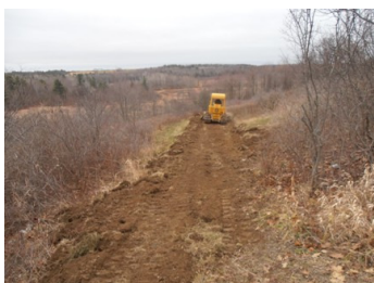
On the south side of Pannis Road another side hill slope is leveled.
