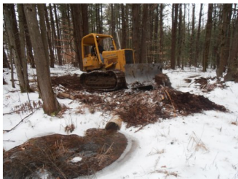
Karl Pritchard works the dirt over a culvert on C7B near Pannis Road.
