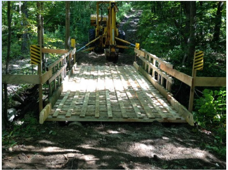
Below is the new bridge, 8' by 25', built and installed by Laudy Hoyenga and his crew.
