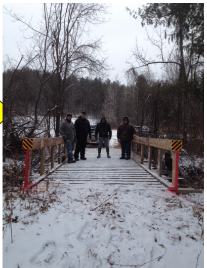
Travis, Chad, PJ Stempel, Brian and Ron doing rail installation on the bridge near Turner Rd. On C7B in East Berne.
