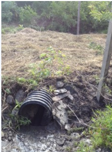
New culvert for Trail S-70 East Berne between Joslyn School Rd and Brookhaven Drive. Photo by Brian Buchardt.
