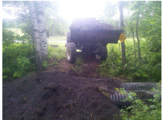
Installing culverts C7B-Knox
