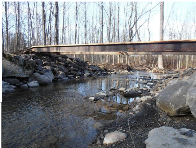
Bridge building C7E-Esperance
